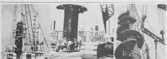
IT TOOK three cranes, skilled operators and capable workmen to erect the seventy-one-foot high tower at AAR-1. The former High Octane Plant tower has been reworked for its new assignment to debutanize in the alkylation complex. A TUMA tres-pro, operadonan experto trahadonan capabel pa instala e columna di setenta-y-un pie alto na AAR-1. E columna anterior Plant ta bini rework pa su nuevo asignacion pa debutanize en el alkylation complex.
